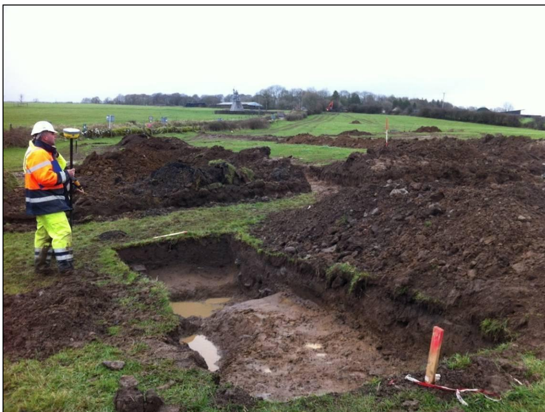
Plate 14.24 Test Excavation in Progress at Shankill
